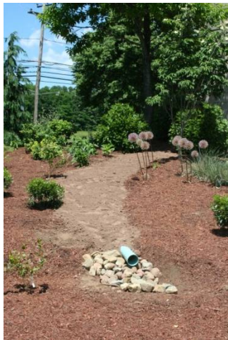
Roof Runoff from Downspout Directed into Rain Garden
